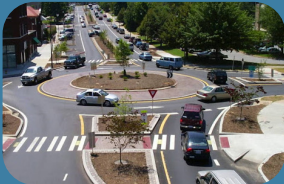
Roundabouts and traffic circles
