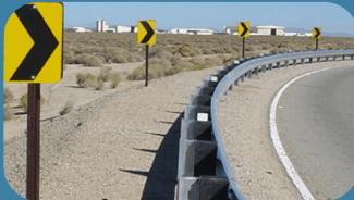
Roadside design improvements at curves
