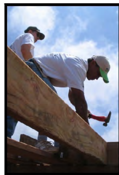
Habitat for Humanity uses donated materials, and the future homeowners help participate in the construction.
