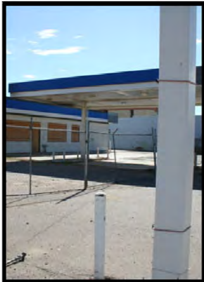
Vacant industrial sites in the Animas district may require environmental remediation.
